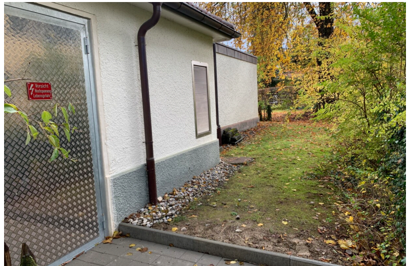
Brunnadernrain transformer station after renovation
