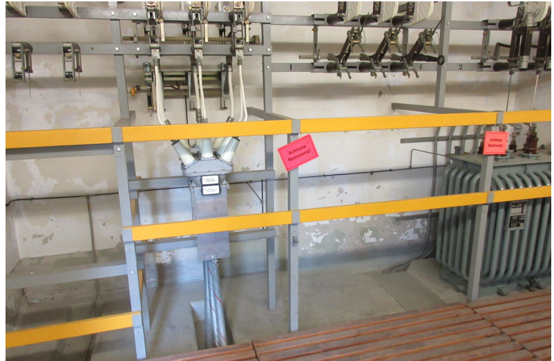
Brunnadernrain transformer station before renovation
